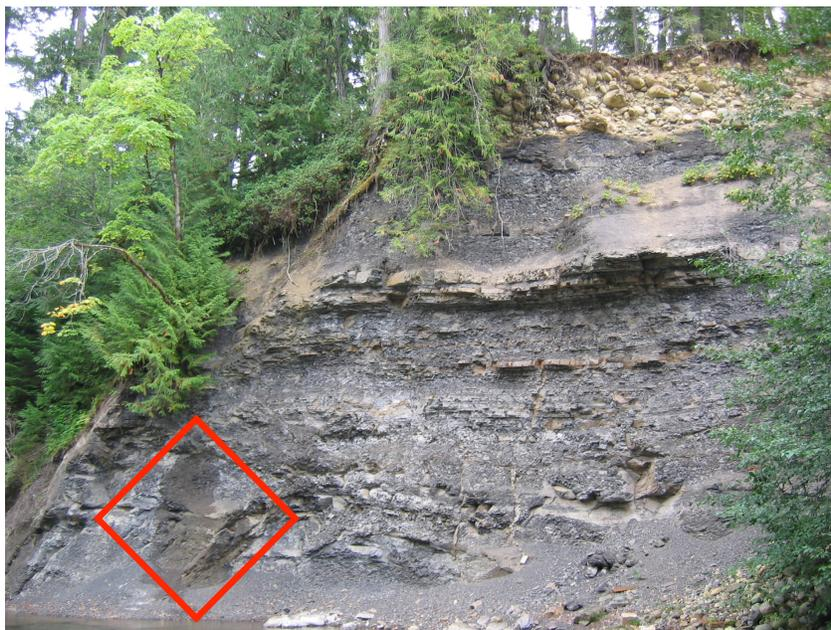
**Figure 10: Seepage on bedrock face (right bank, 15.9 km)**
