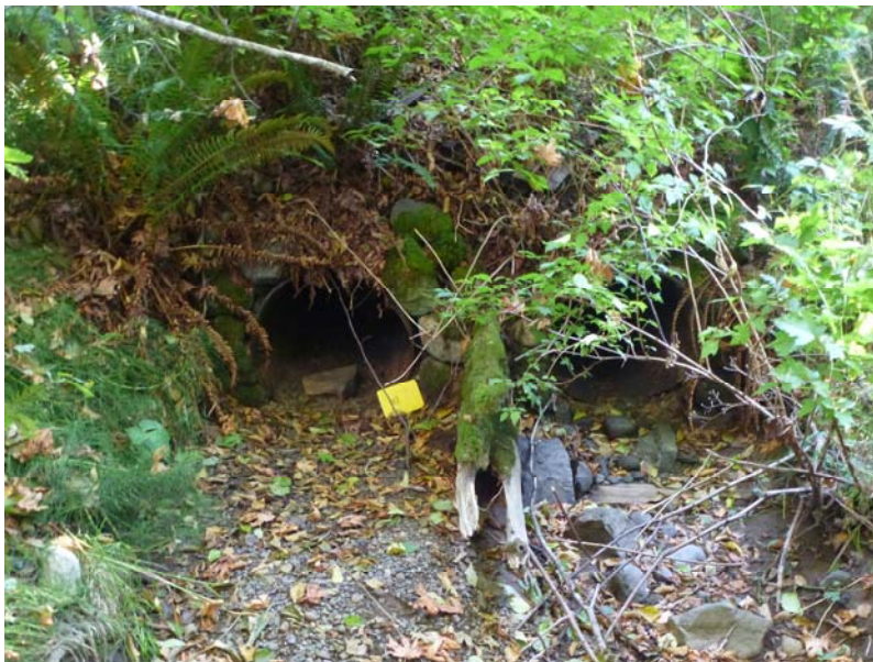
Photo 16. Upstream view towards culverts crossing under the railway
