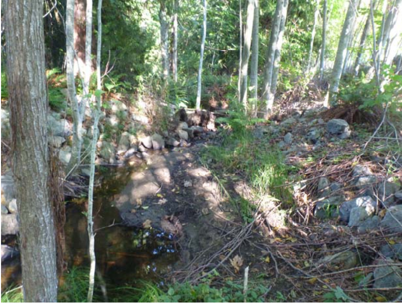
Photo 13. Downstream view of Shelly Creek between storm drain and Hamilton Avenue
