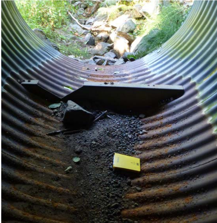
Photo 17. Downstream view from inside the Wildgreen Way culvert
